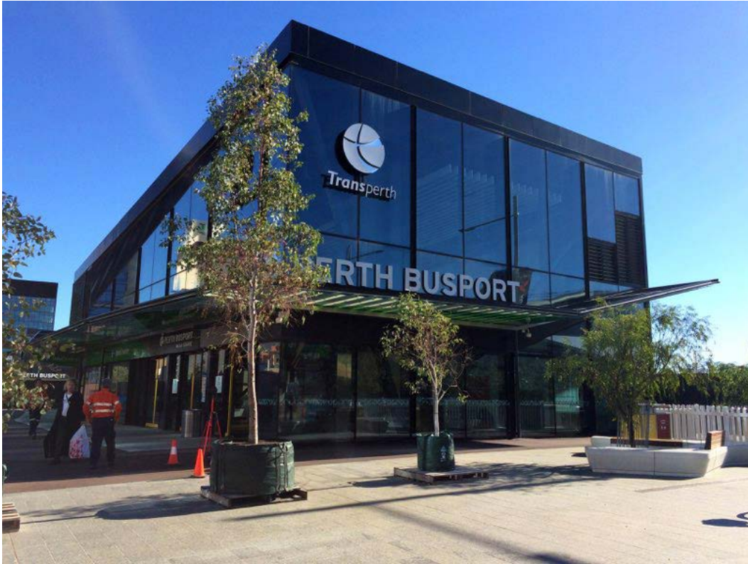
Figure 2 Main Entrance to the Perth Busport
